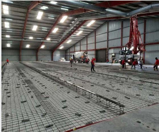
BANAIR® full turn-key/ground preparation for a large mobile based ROLLINGSTACK project in Sanem, Luxembourg. (See case study)
